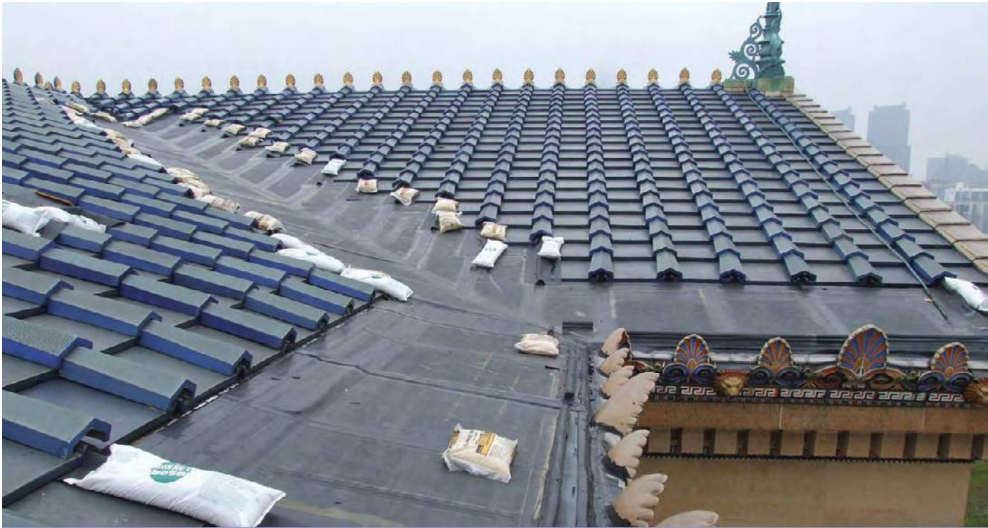
The flashing work in progress. Photo courtesy of LF Driscoll.
