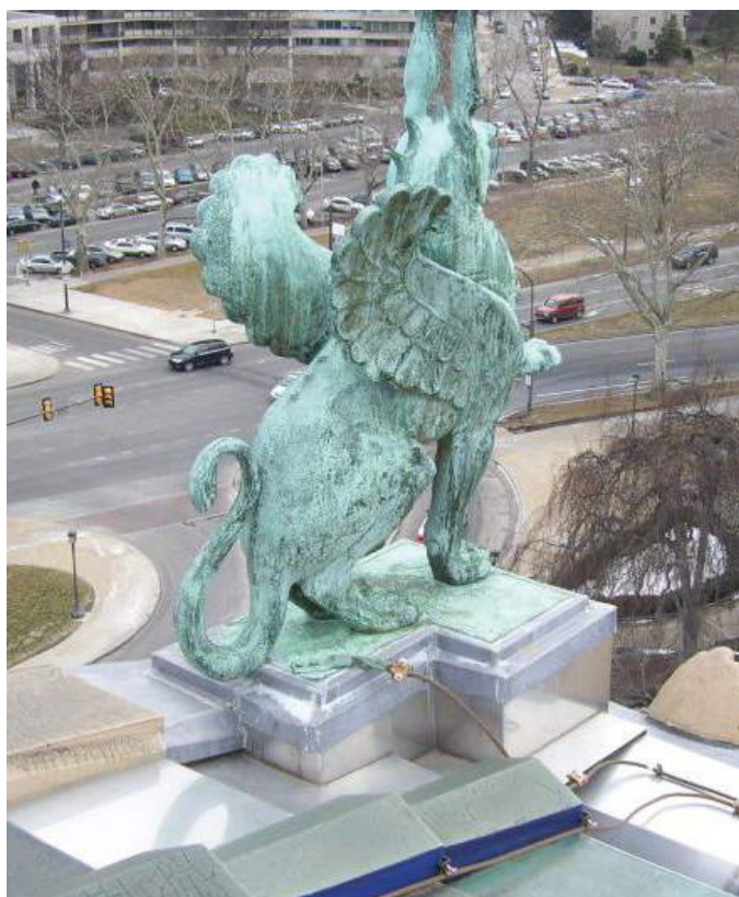
The bronze griffin protects the Museum by safely conducting lightning strikes into the ground via copper cables that are UL-listed for use in lightning protection systems. Photo courtesy of Warren Lightning Rod Co.
