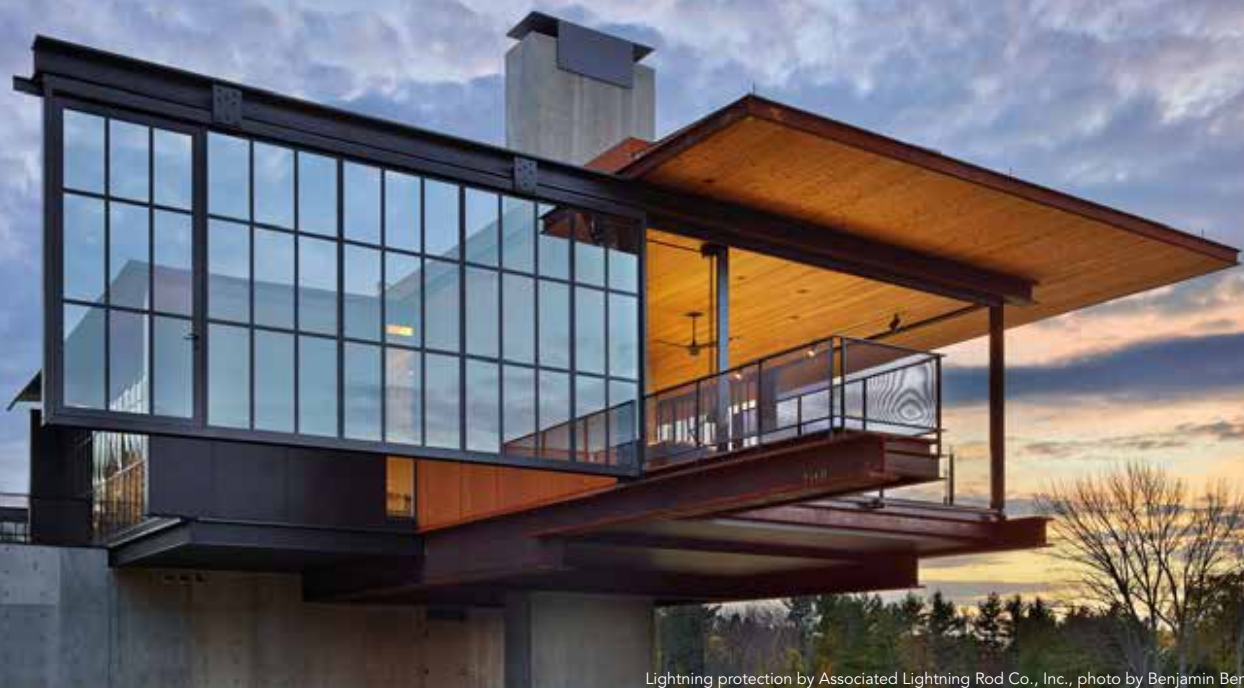
Lightning protection by Associated Lightning Rod Co., Inc., photo by Benjamin Benschneider
