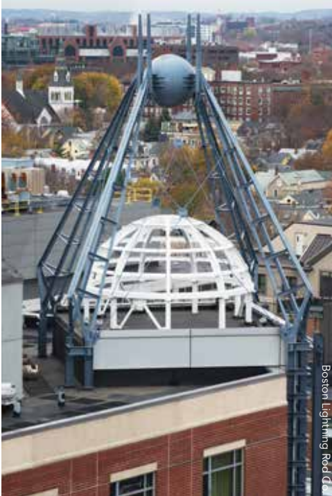
▲ The steel turret atop Le Méridien-MIT Hotel in Cambridge, Mass., acts as a strike-termination device and is connected via the LPS to ground. A conventional air terminal is visible on the parapet in the lower-left corner of the left photo.
