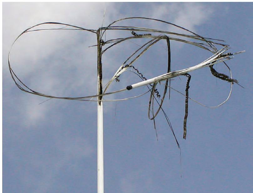
Figure 4 — Lightning destroyed this antenna. A properly designed and installed lightning protection system could have prevented this damage and provided protection for the owner’s home and its contents.
