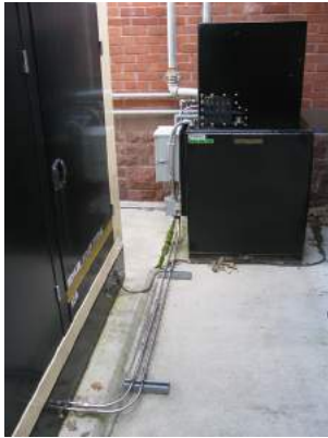
Figure 5. Grounding connection to the station's emergency generator shown at left. The braided bare copper grounding cable used here is routed to the generator fuel tank, center, and thence to the station grounding system via a wall penetration visible at right rear.
