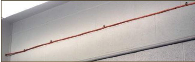
Figure 10. Upper photo: grounding conductors run along walls and from room to room in the venerable fire station. Lower photo: a copper ground bar serves as the ground-to-lightning system bus at the station's service entrance. Note that braided copper lightning cable extends all the way to the service entrance.
