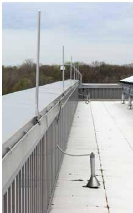
**Figure 2:** Air terminals are mounted on the back of a parapet to minimize visibility; conductors lead to through-roof penetrations.
